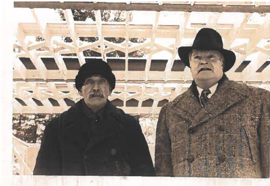
The builder, Fred Booth, and the designer, Henri Pontbriand—the second clubhouse under construction
